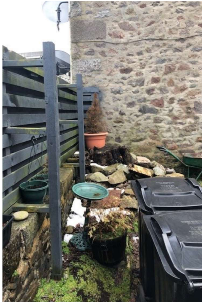
Existing fence/wall (facing south)
